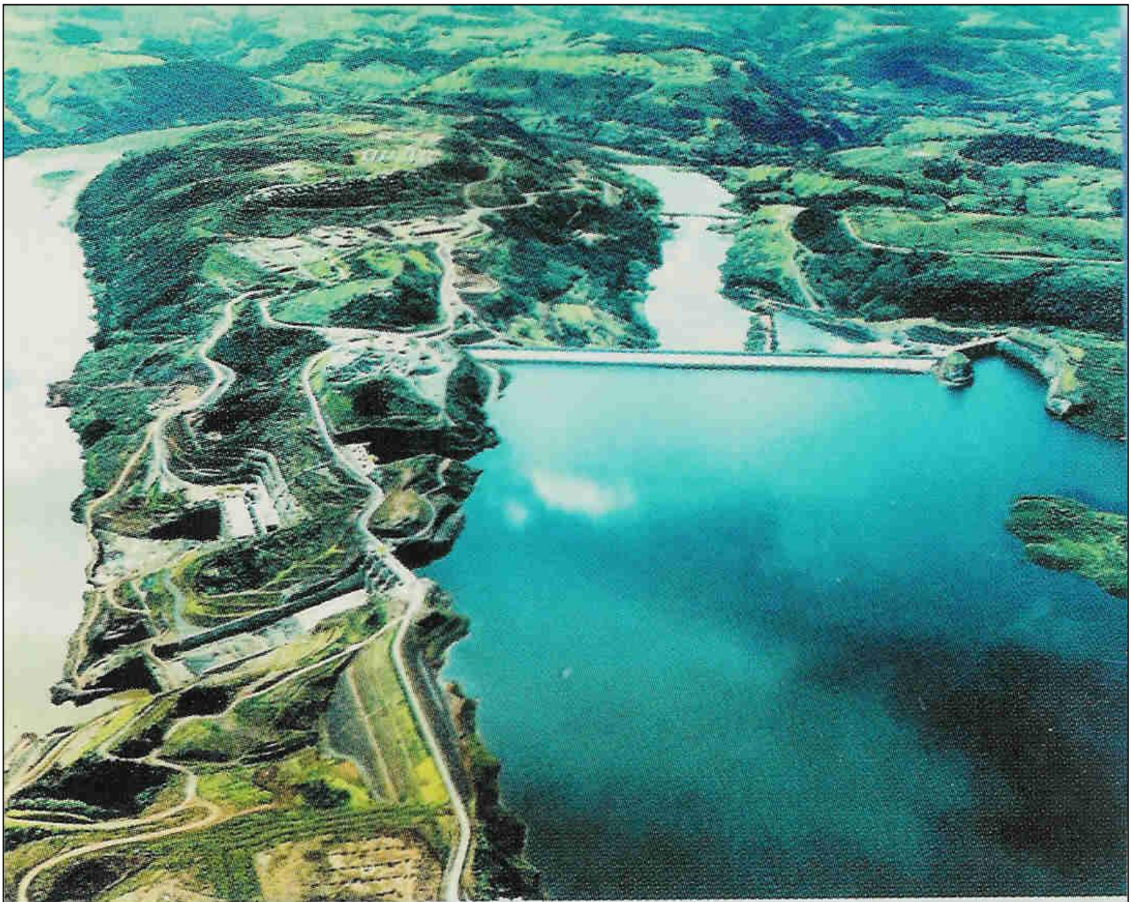
The 125 m-high Itá concrete-faced rockfill dam and 1450 MW powerplant in Brazil
